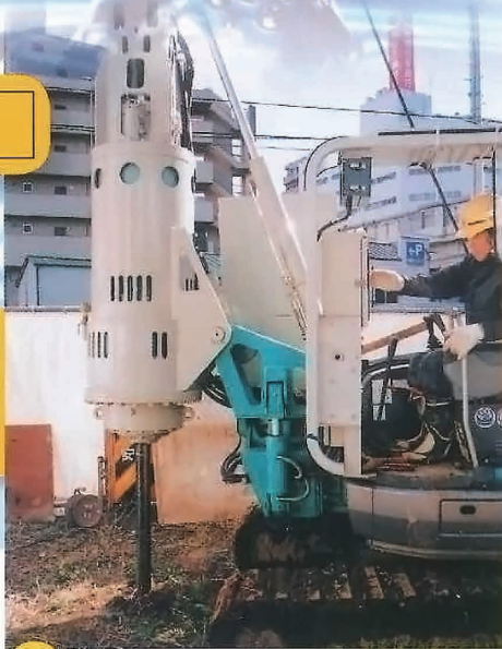
1 purification works by a boring machine
