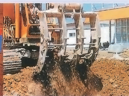
mixing fork Removes the rocks in the soil before application and mixes the soil and the purification liquid after application
